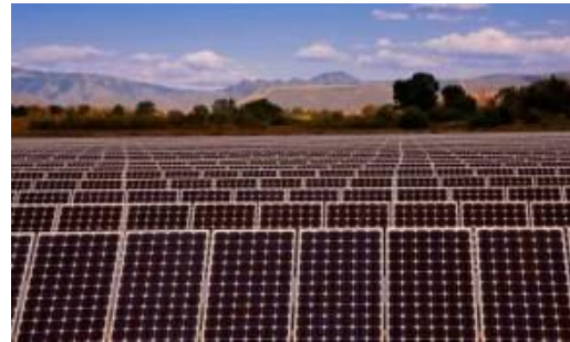
Fig.2: Solar Generation Unit
